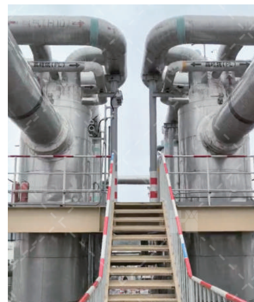
新能源行业用绕管式热交换器 Spiral wound tube heat exchanger for new energy
