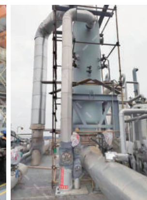
三管板循环气预热器 DN1400×4500mm Circulating gas preheater with 3 tube sheets
